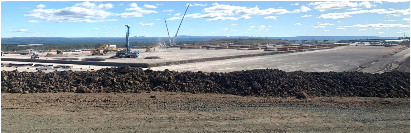
Construction at Oakdale West
