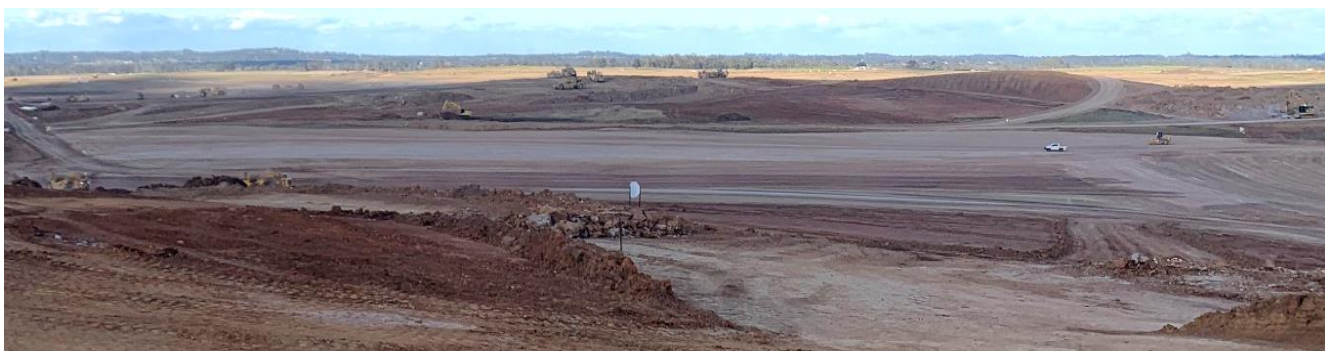
Scrapers working to move 25 million cubic metres of earth at the new airport
